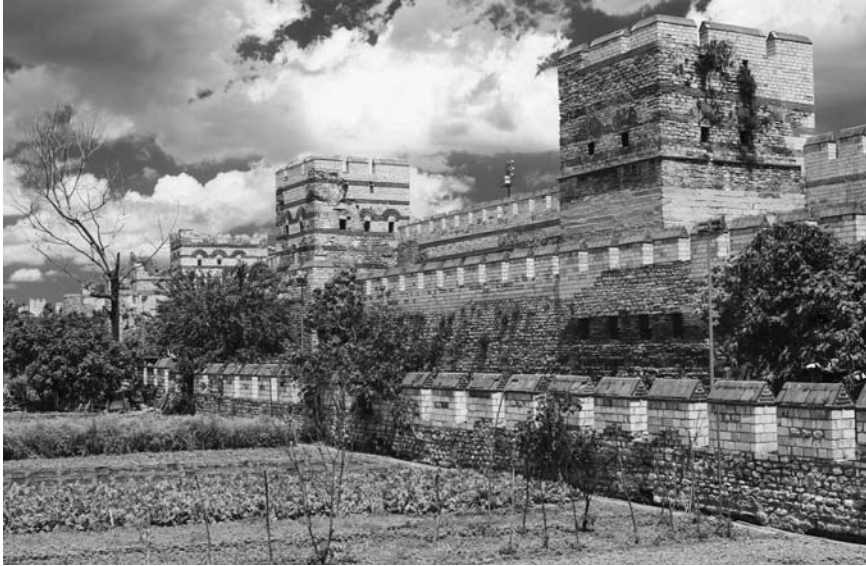
FIGURE 1 The Land Walls of Constantinople, as recently restored, showing the outer and inner walls, some of the 96 defensive towers and the site of the moat, now occupied by vegetable plots. (Vlacheslav Lopatin/Shutterstock.com)
